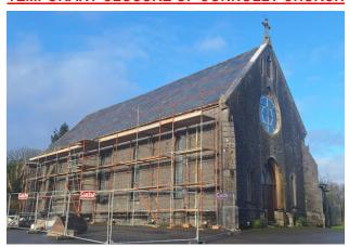
In order to facilitate works to replace the roof in Connolly Church, it is necessary to close the church until the project is complete. The project involves, stripping the roof, adding insulation and new felt and covering it with replacement slates. The cast iron downpipes and gutters will also be restored. We are at the mercy of the weather but hope to be back in the church for Christmas.
